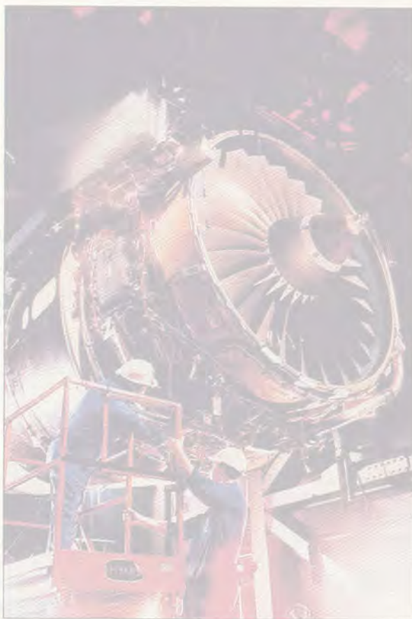
The Rolls-Royce test cell is being built to test the 70,000-lb. thrust Trent version of the RB211.
